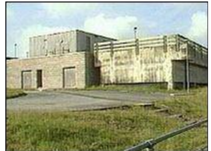
Lowermoor water works. ( http://news.bbc.co.uk/2/hi/uk_news/england/cornwall/7142515.stm )
