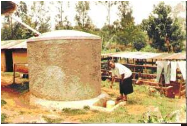
A mother fetching water from a ferro-cement tank constructed by RSP. ( www.rspkaimosi.org )
